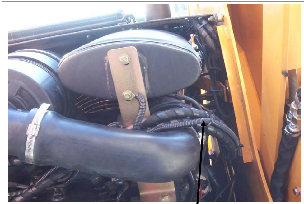
A/C lines and electrical ground wire coming from condenser.
